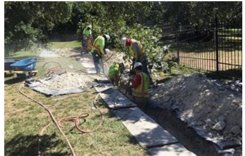
Underground rehab in progress
