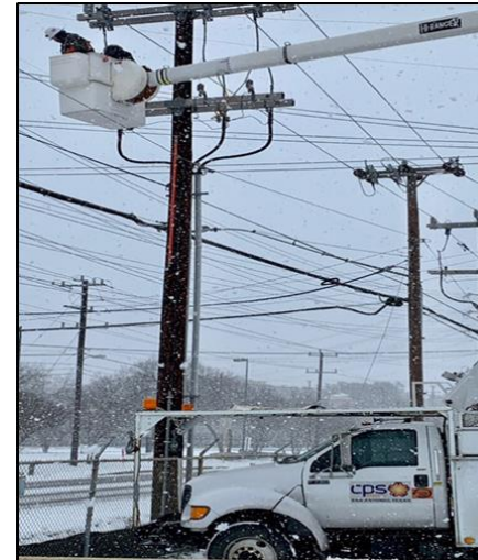
Repairs During Winter Storm
