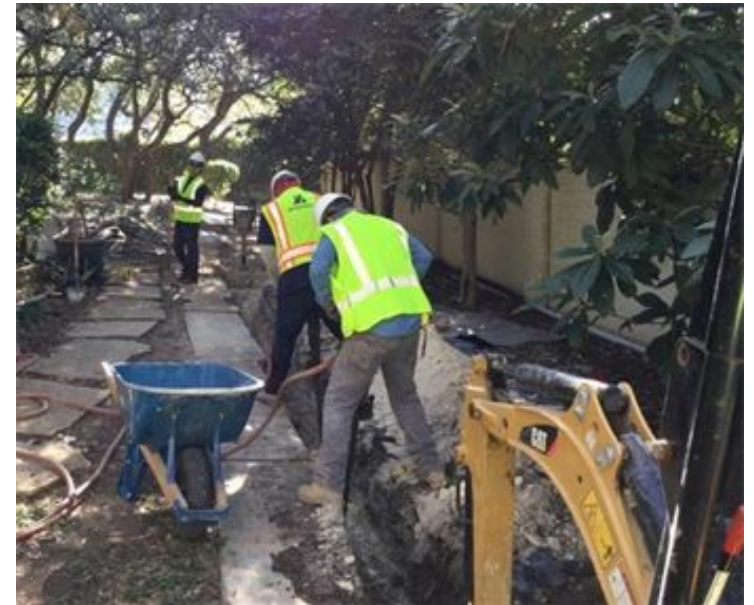
Underground rehab in progress
