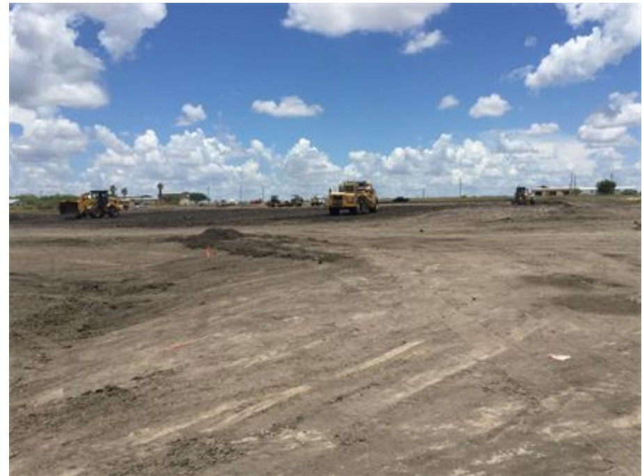
Site work & grading for a new substation
