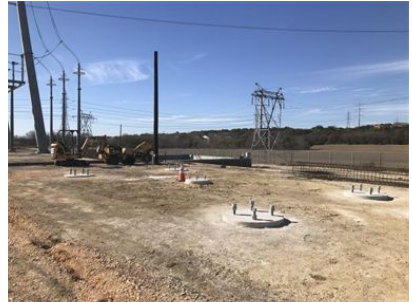
Installation of new foundations
