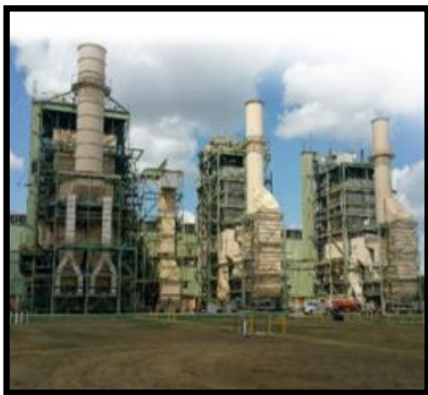
Braunig Gas Power Plants were built in the late 1960s
