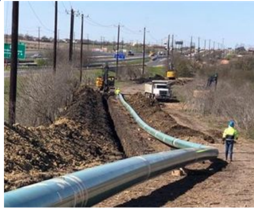
Gas Main Construction
